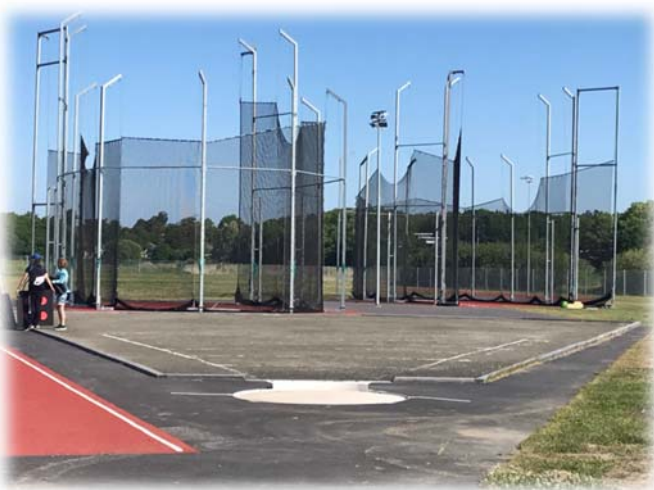
The brand new Bjorlanda Stadium will provide throwers with excellent facilities.
